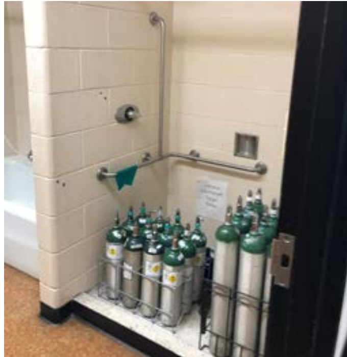
Oxygen tank storage in a shower stall in a Colerain Elementary restroom
